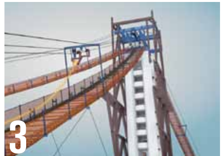
3 Strand is hauled over the Tower Cable Saddle
