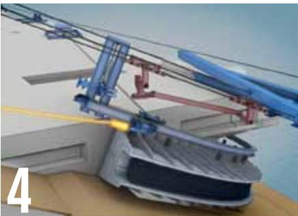
4 Strand reaches west end and is attached to secondary hauling system
