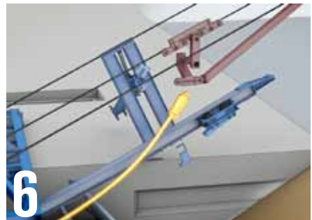
6 Strand is re-attached to primary hauling system and is pulled up and over the tower to the east end of the eastbound deck
