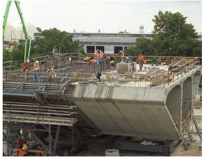
Segments being match cast to ensure a perfect fit.
