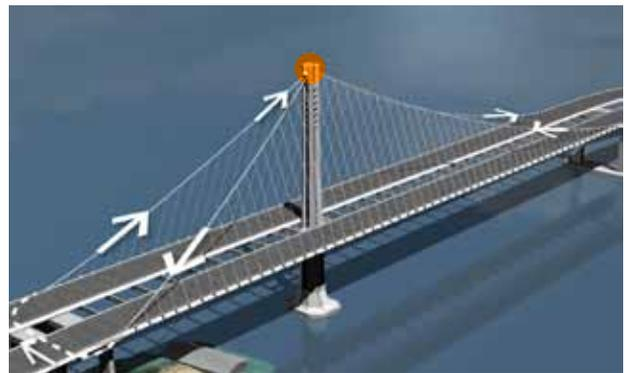
The tower will be complete after the cable is placed and the tower head is attached.
