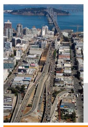
As part of this \$429 million retrofit-by-replacement project to rebuild the West Approach, the double-deck roadways from 3rd Street to the anchorage are being rebuilt so that each deck will have independent columns and foundations.
